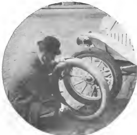
Fig. 1—First operation in adjusting Jenkins Emergency Wheel
